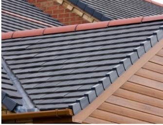
**Roof.** You don't need to climb up there yourself; with binoculars and a keen eye, you can probably spot trouble. Do you see any shingle-shift, suggesting that some fasteners may have failed and need replacing? Any cracked or missing shingles? What about
