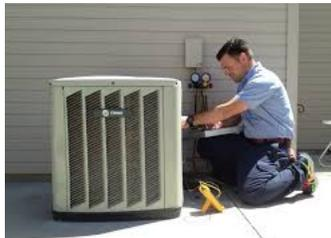
**Air Conditioning.** Just as you readied your furnace for fall, now is the time to make sure that air conditioning units are in good working order for the warmer months ahead. Change the filter, check hose connections for leaks, and make sure the drain pans are draining freely. In addition,
