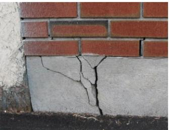
**Foundations.** When inspecting the exterior of your home, be sure to examine the foundation from top to bottom for masonry cracks. "Routine caulking by homeowners won't do the job," says Niles. "Hire a foundation specialist who can employ a two-part epoxy
